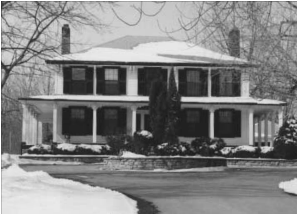
◀ Italianate. The Grange , located on Burns Place, boasts wide eaves and a sloping hip roof, characteristic of its current Italianate style.
